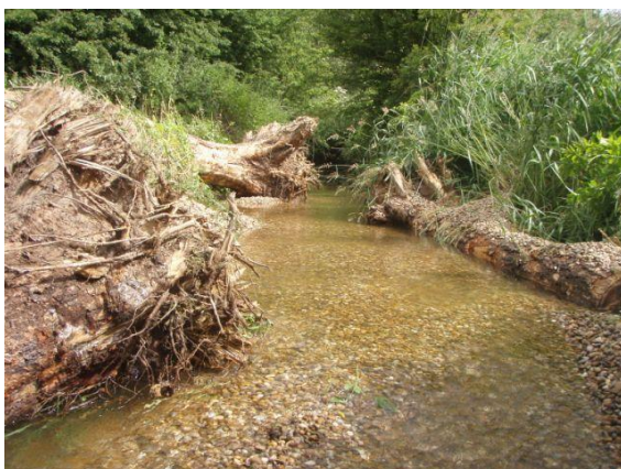
Figure 5 Large woody debris placed along river banks
