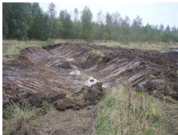
Figure 8 New meander being excavated
