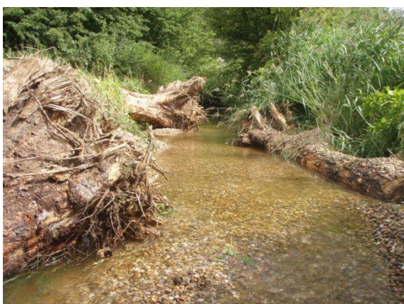
Figure 5 Large woody debris placed along river banks
