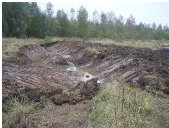
Figure 8 New meander being excavated
