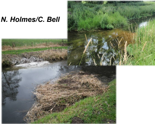
Figure 5: Double berm under construction (left, far bank berm yet to be capped) and 4 months later (right)
