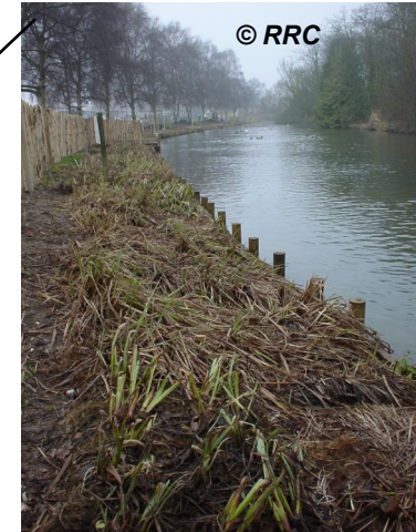
4. River Wensum at Fakenham Soft revetment works (Figure 6).
