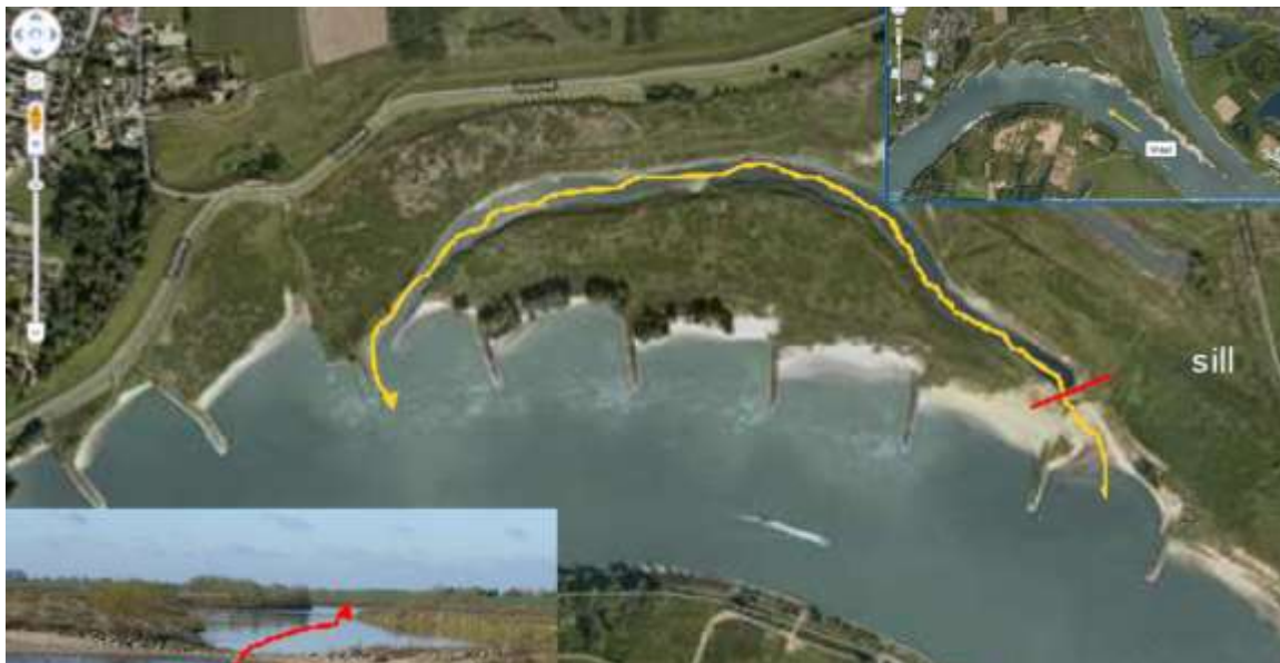
Figure 1 – A photograph (post-project) of the dyke relocation at Klompewaard. The inset picture shows the direction of the flow of the River Waal through this section.
