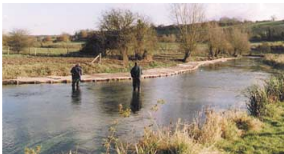
Demonstration site ledge – just completed
