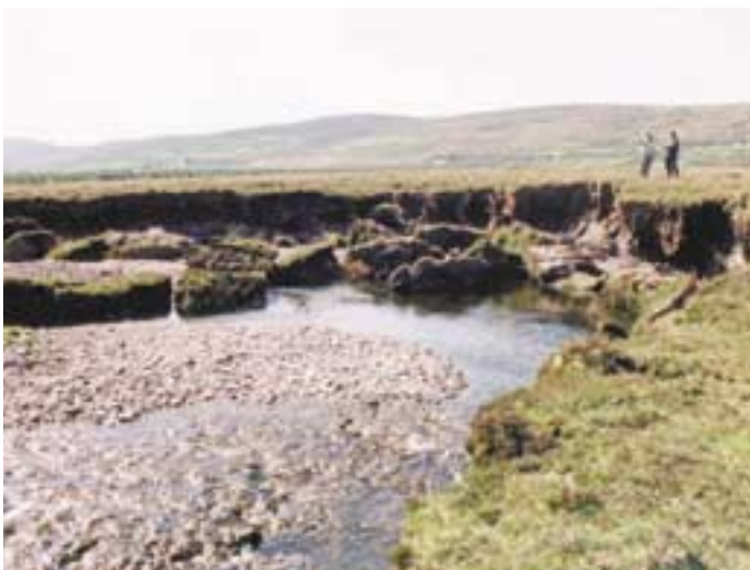
Over-active erosion of banks. Eroding channel due to bank instability.
