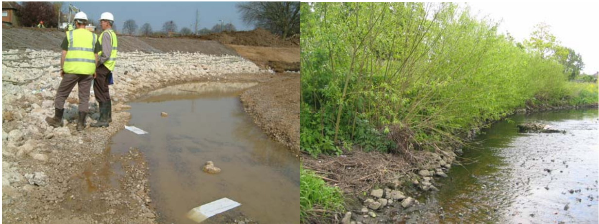
The crushed concrete protection being installed, and two years later with the willow growth.
